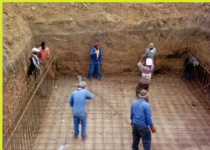
Construction of ABR for institutions and settlements
