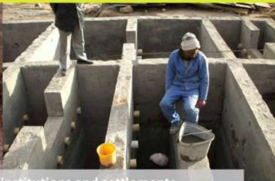
Construction of ABR for institutions and settlements
