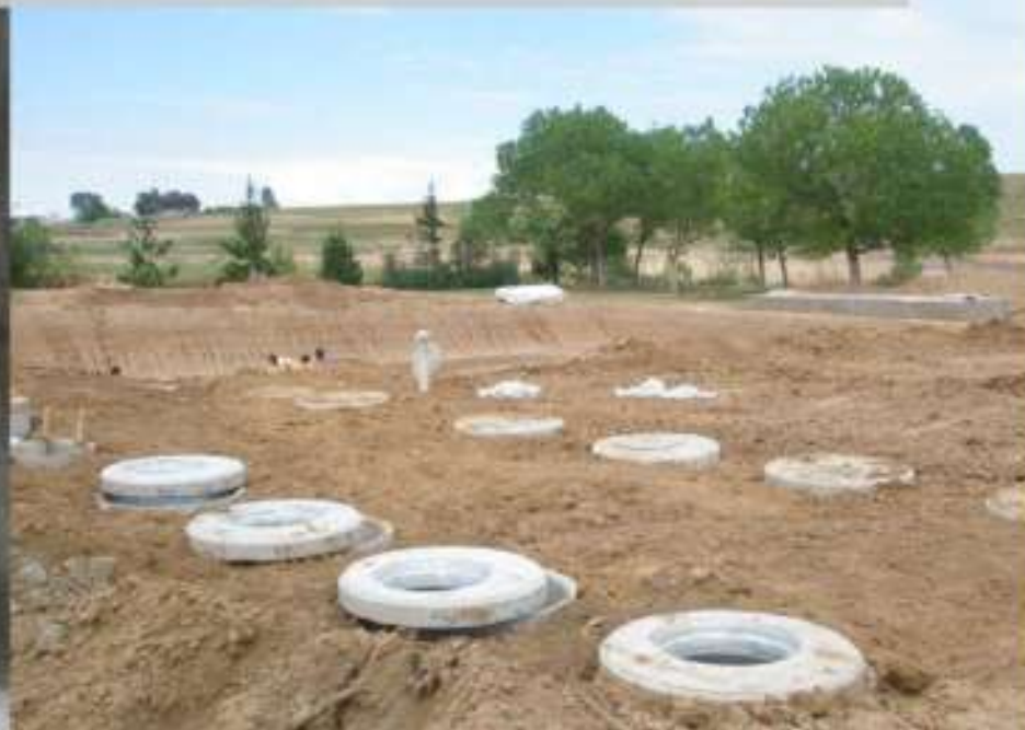
Construction of ABR for institutions and settlements
