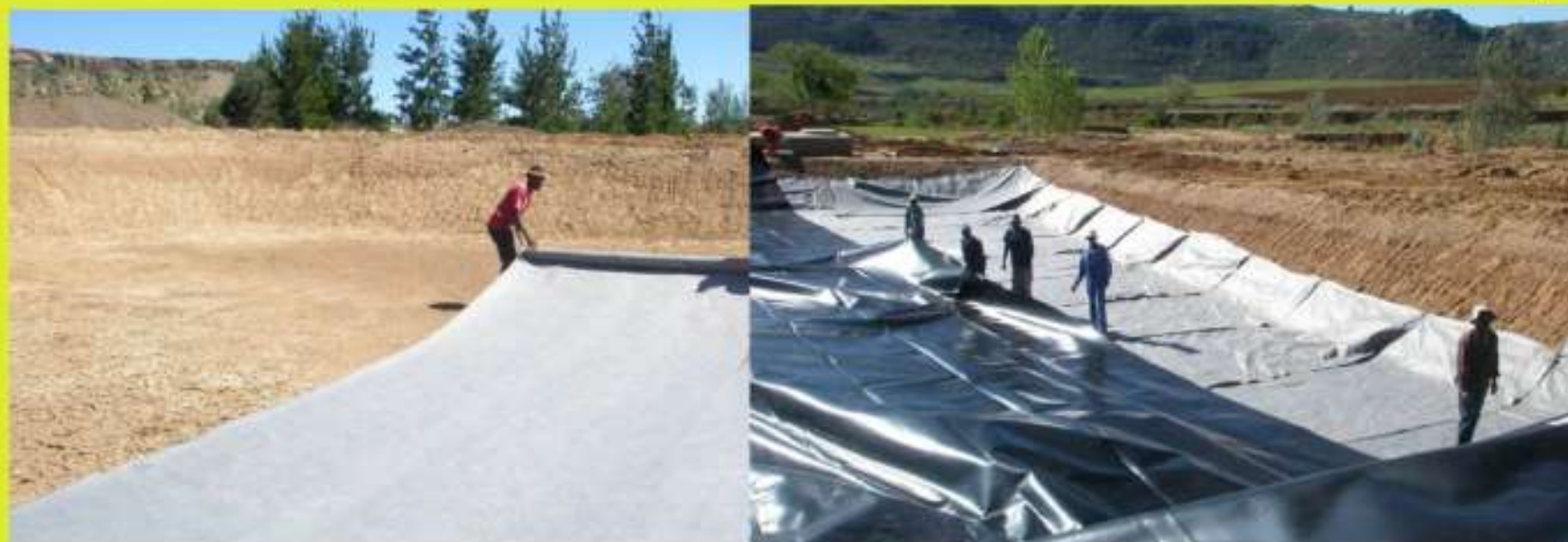
Construction of horizontal filter (PGF) for institutions and settlements
