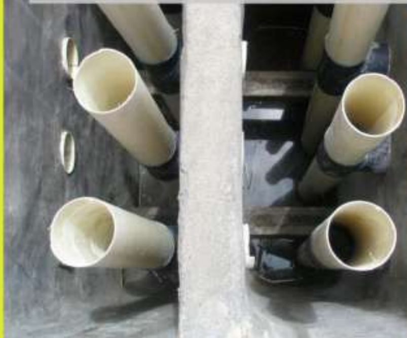
Construction of ABR for institutions and settlements
